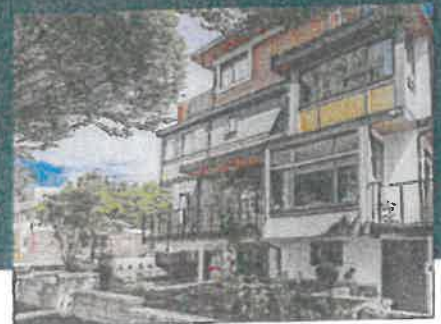
Small-scale multifamily building
