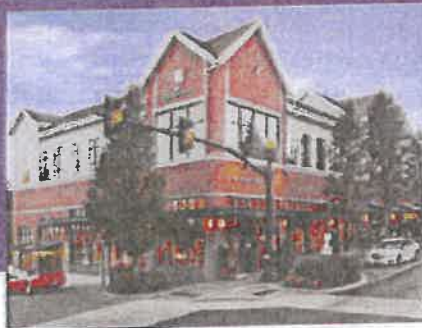
Retail/commercial building on main street corner
