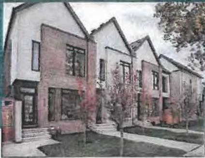
Townhouse cluster along a public sidewalk
