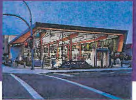
Retail building with high quality street frontage
