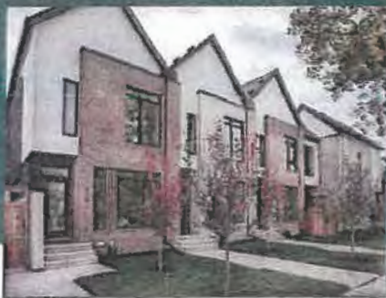
Townhouse cluster along a public sidewalk
