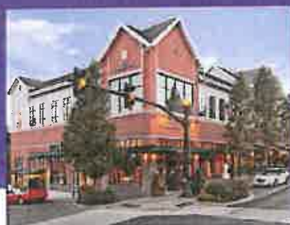
Retail/commercial building on main street corner
