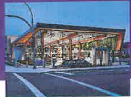
Retail building with high quality street frontage
