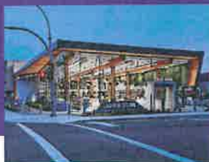
Retail building with high quality street frontage
