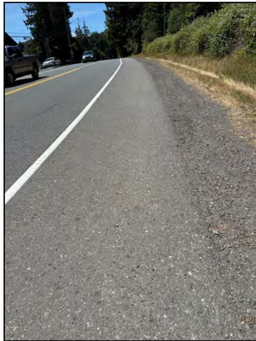
Road Shoulder, 1.5 m asphalt
