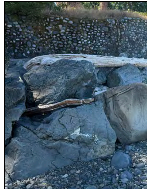
Old concrete/stone wall and rip rap.
