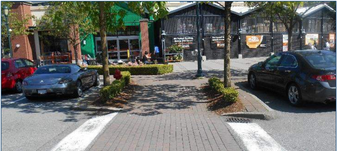
Figure 41: Curb extension and raised crosswalk.
