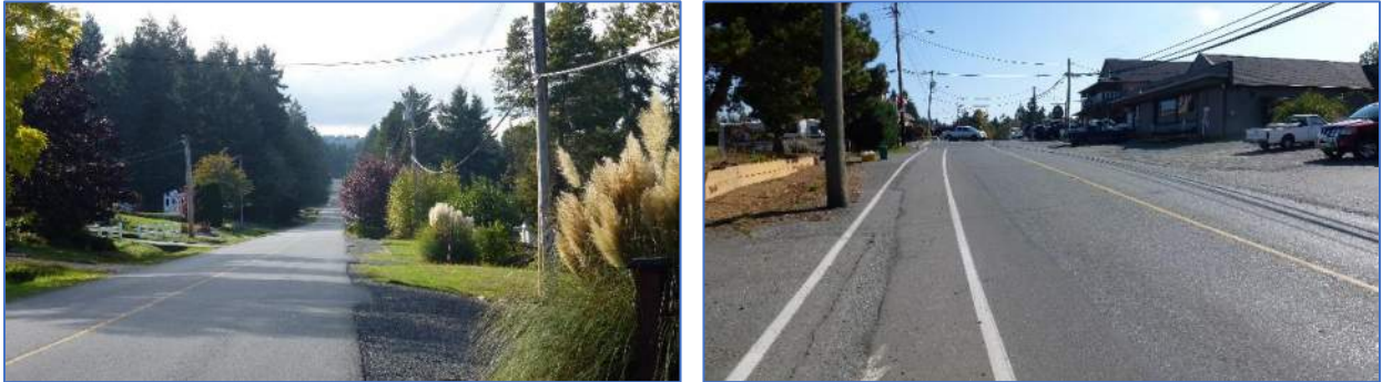
Figure 14: Roads in Lantzville are built to a rural standard, without curb and gutter or sidewalks (left), Painted pedestrian areas and raised crosswalks have been recently added to the Village to increase safety, but parking and pedestrian conflicts remain (right).
