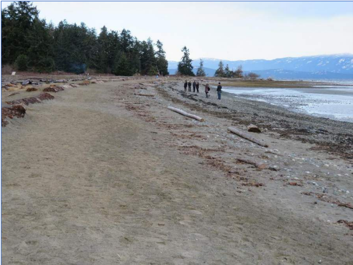
Figure 57: At Rath Trevor Provincial Park, a seawall causing waterfront erosion was replaced by beach nourishment sands and gravels in a "Green Shore" approach
