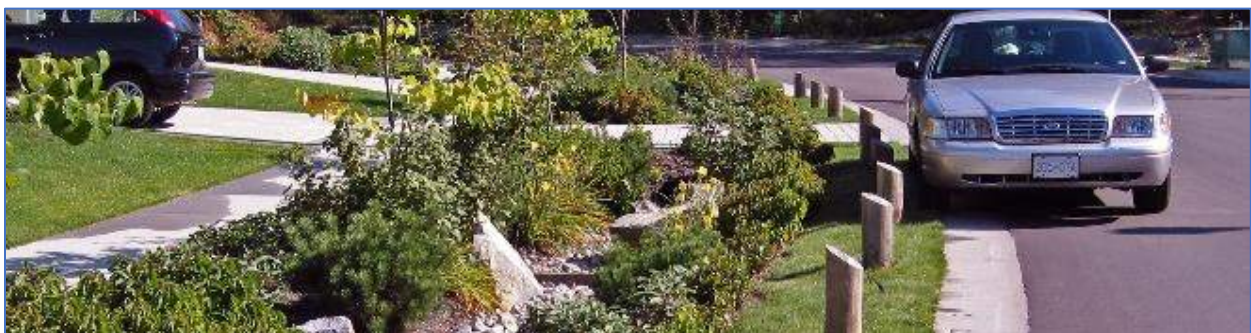
Figure 21: Storm water source controls – infiltration swale.
