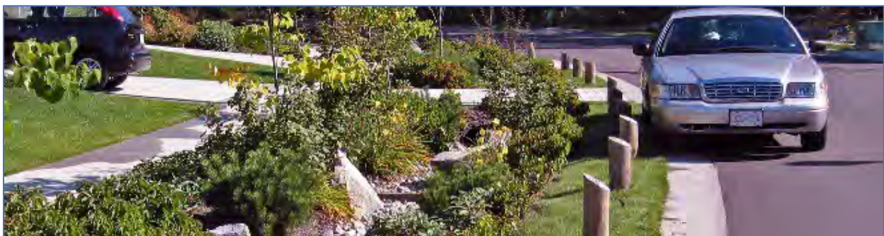
Figure 21: Storm water source controls – infiltration swale.
