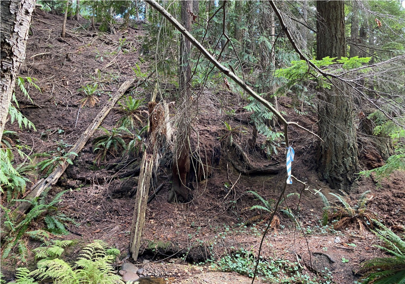
Photo 2.2.1 – Watercourse bank conditions on 6852 Wiles Road, looking west.
