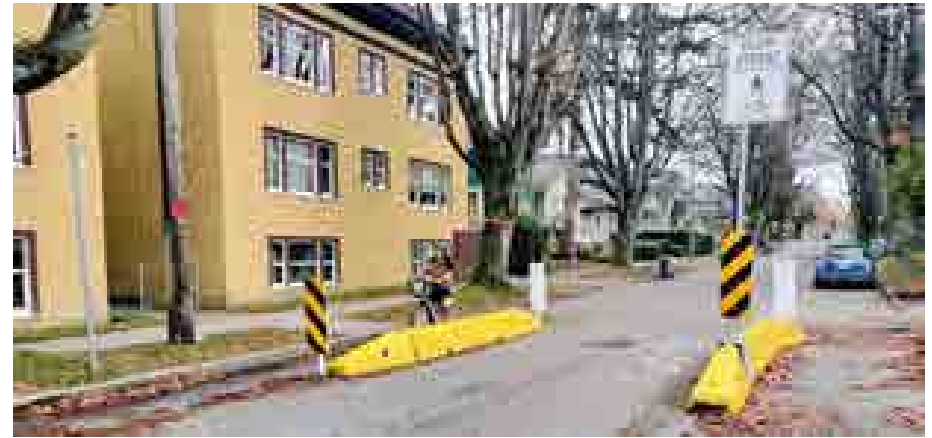
Example of slow street barriers in the City of Vancouver. The barriers create a gateway to encourage drivers travelling at higher speeds on major streets to slow down as they enter the neighbourhood. Image credit: City of Vancouver
