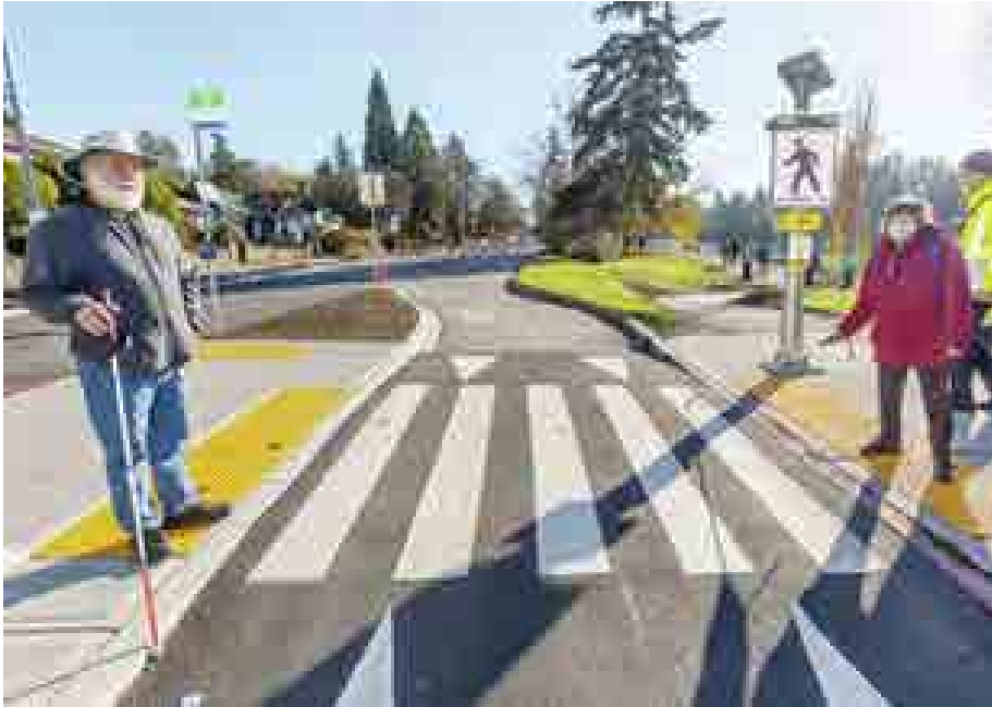
Example of a raised crosswalk featuring tactile paving to alert vision-impaired users that they are entering a curb ramp, as well as rapid flashing beacons to alert drivers that a crossing is taking place. Image credit: Times Colonist
