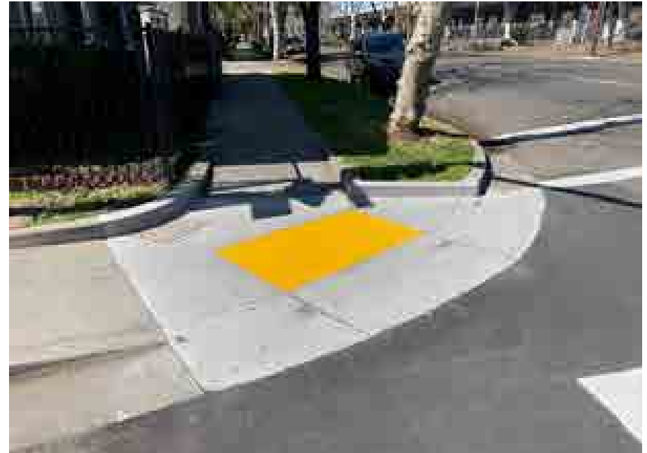
Example of a curb ramp with a tactile surface to alert vision-impaired users. Image credit: City of Sacramento
