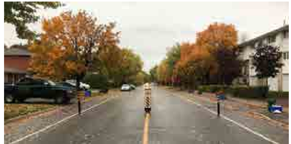
Example of flex stakes (flexible bollards) in the City of Greater Sudbury. Image credit: City of Greater Sudbury
