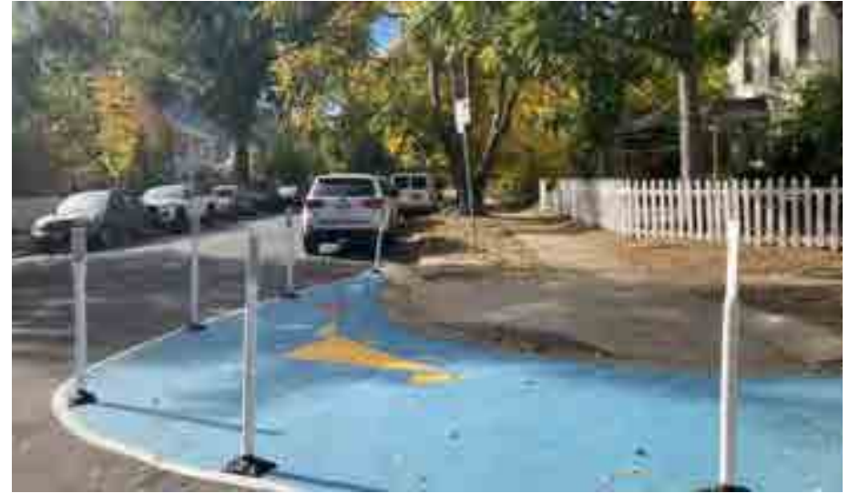
Example of a quick-build curb extension in Boulder, Colorado. Image credit: City of Boulder
