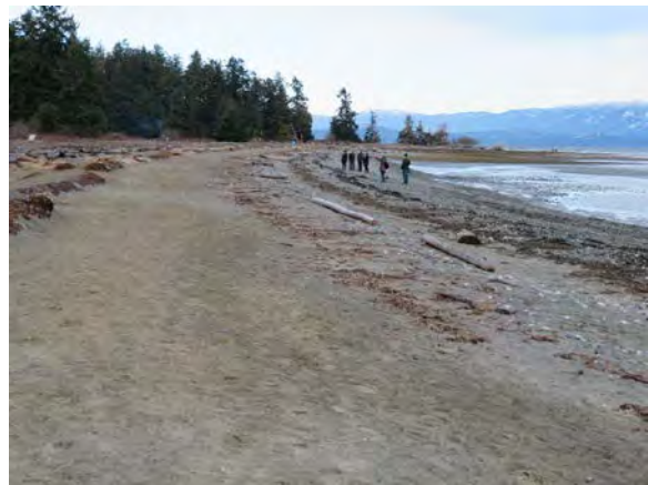
Figure 80: At Rath Trevor Provincial Park, a seawall causing waterfront erosion was replaced by beach nourishment sands and gravels in a "Green Shores" approach
