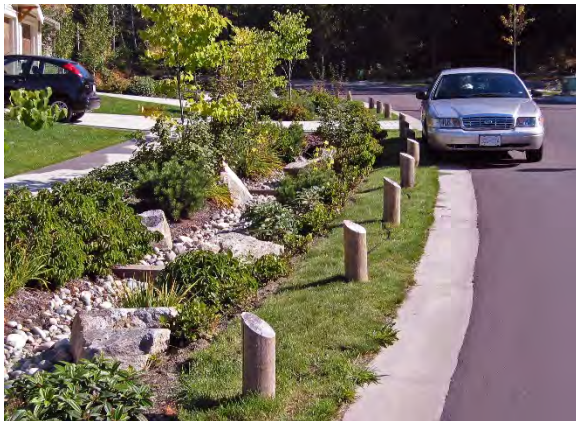
Figure 35: Storm water source controls – infiltration swale
