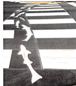
New crosswalks in Tofino feature a fish motif
