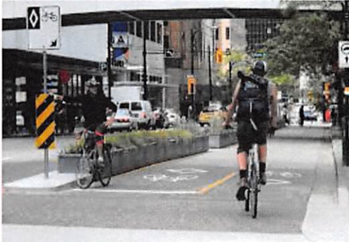
Planter boxes delineate a new bike lane in Vancouver. This is an example of the kind of tools that could be used to delineate pedestrian areas.
