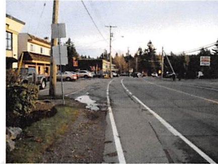
The pedestrian lane on the north side of Lantzville Road is currently painted in. This approach could be replicated in the shorter term, to outline a pedestrian area, but relocated to the outside of the road right of way, with on-street parking further to the inside.
