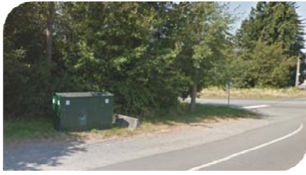
Ware Road Pressure Reducing Valve (2000)
